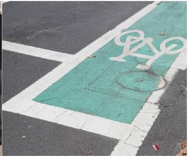
Photo 4.2: Bicycle head start box at traffic signals
